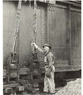
Open hearth, Port Kembla steelworks. Rigger slinging an 85-ton girder. Photograph by T.S. Fisher, July 1938.
